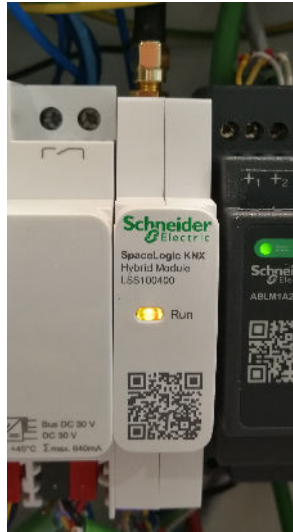
Hybrid Module in the cabinet
