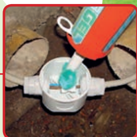
UNDERGROUND CONNECTIONS
