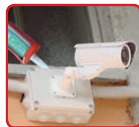
CONNECTIONS IN MOIST ENVIRONMENTS
