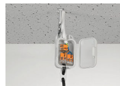
Pendant light connection in a suspended ceiling
