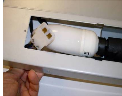
Figure 8: Passing cable through
